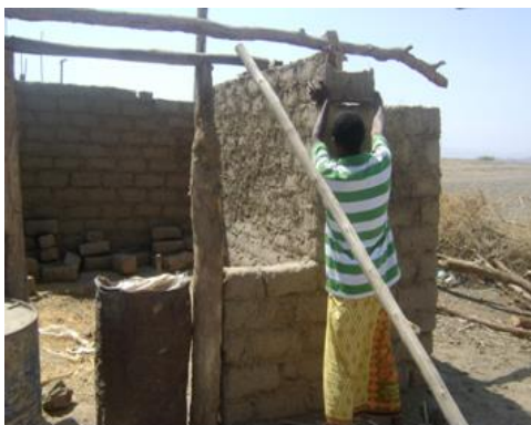
Working on Mud-block house construction - Awra
