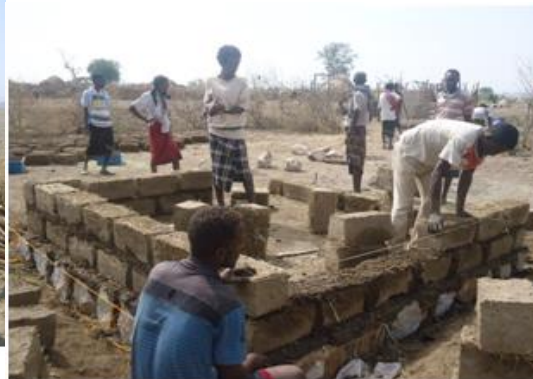
Working on Mud-block house construction - Awra
